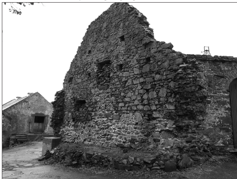
Pl 2 Exterior of gable 1. Note the sandstone sill in the window and the projecting masonry over what would have been the old road, inspiring the gateway in the reconstruction (Fig 4).
