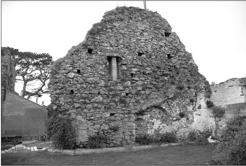
Pl 3 Exterior of gable 2 illustrating blocked doorway and window, both off-centre in the wall.
