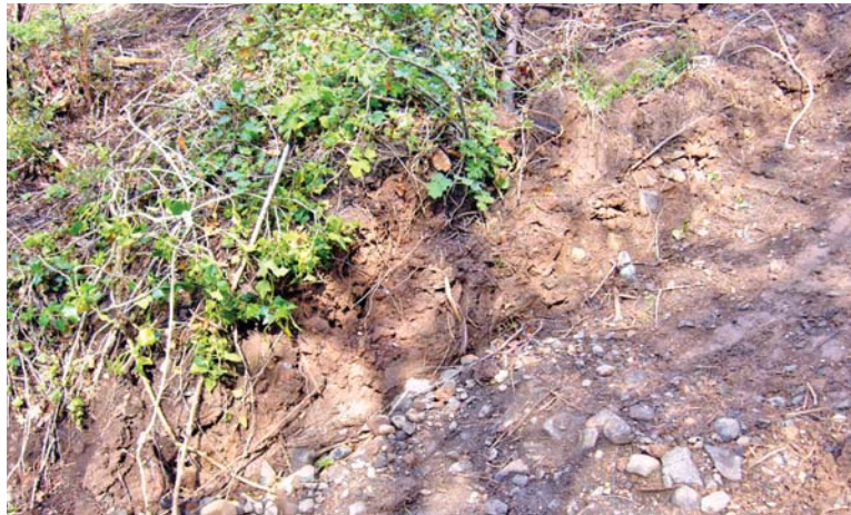
PLATE 17: Bridge Footings 1: detail of depth of excavation of bridge footing
