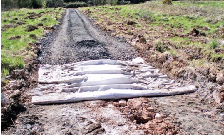
PLATE 7: Section 2: section of partially constructed footpath.
