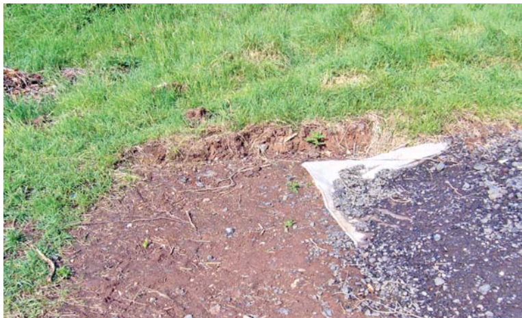
PLATE 2: Section1: Detail of unfinished pathway showing depth of excavation.
