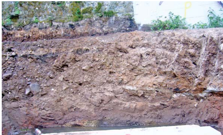
PLATE 24: Bridge Footings 4: bridge footing on south bank of Three Mile Water. Note disturbed nature of ground.
