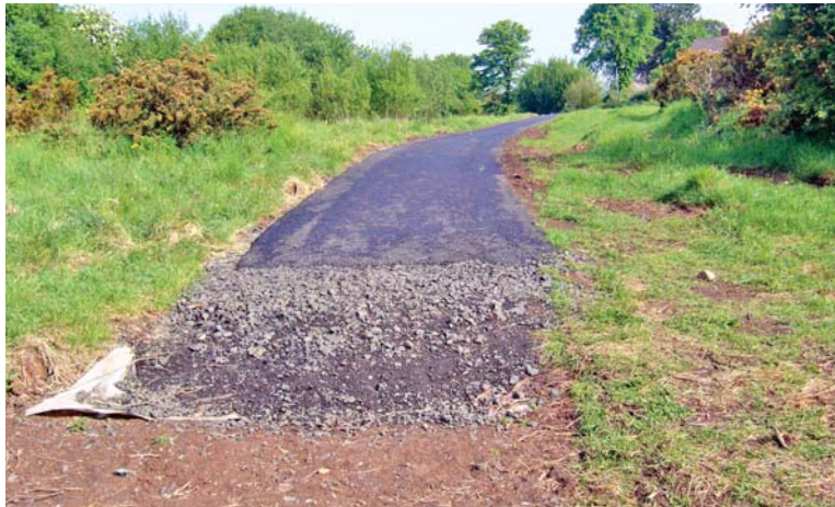
PLATE 1: Section 1: Looking at section of unfinished pathway towards Three Mile Water.
