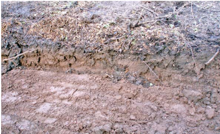
PLATE 14: Section 3: detail of depth of excavation showing glacial subsoil approximately 0.4m below current ground level.
