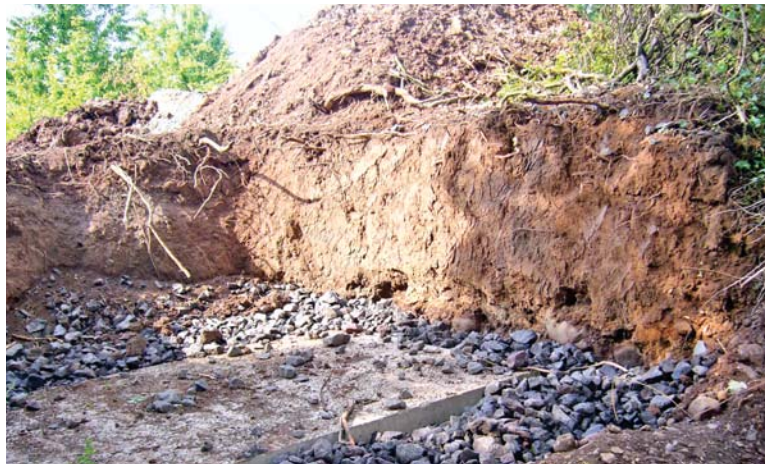
PLATE 18: Bridge Footings 2: bridge footings on south bank of the Three Mile Water. Note clean orange boulder clay comprising section face.
